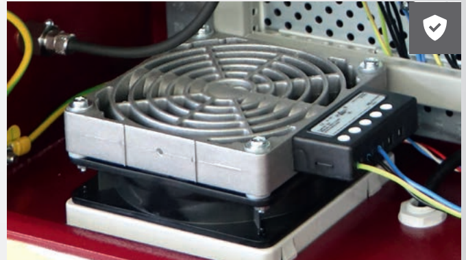
Cabinet heating Temperature regulated, for use in safe environment
